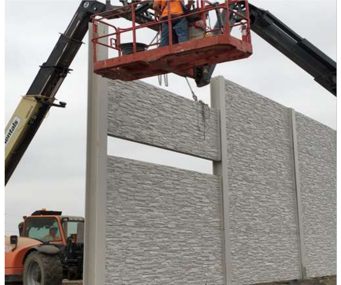
Installing wall for a 20ft high reflective sound barrier wall
