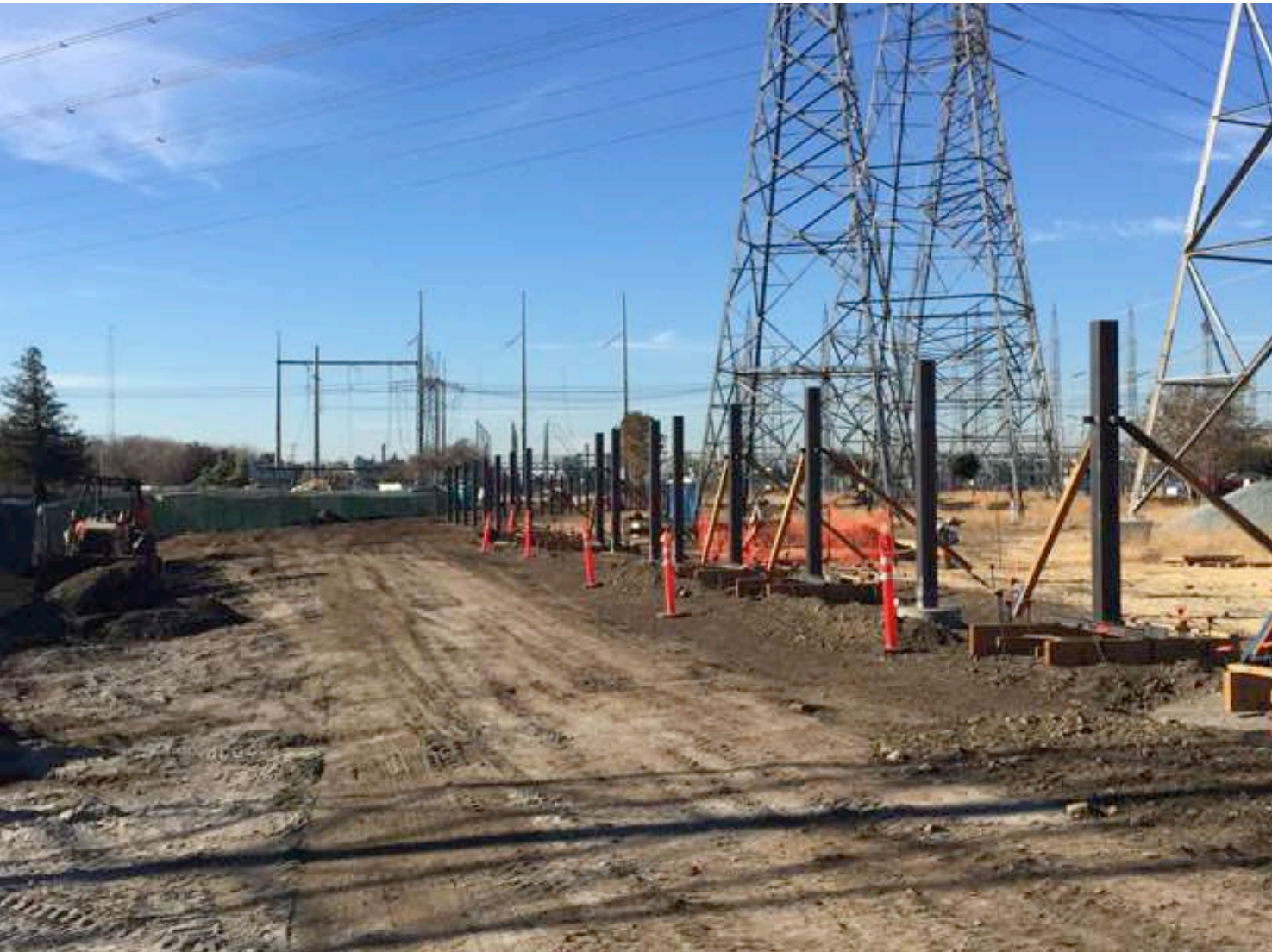
Footings with Extended Steel Supports Are Set Up for Taller Walls
