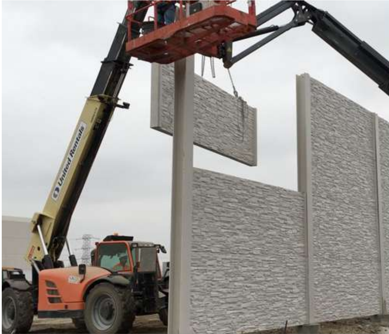
Installing wall for a 20ft high reflective sound barrier wall
