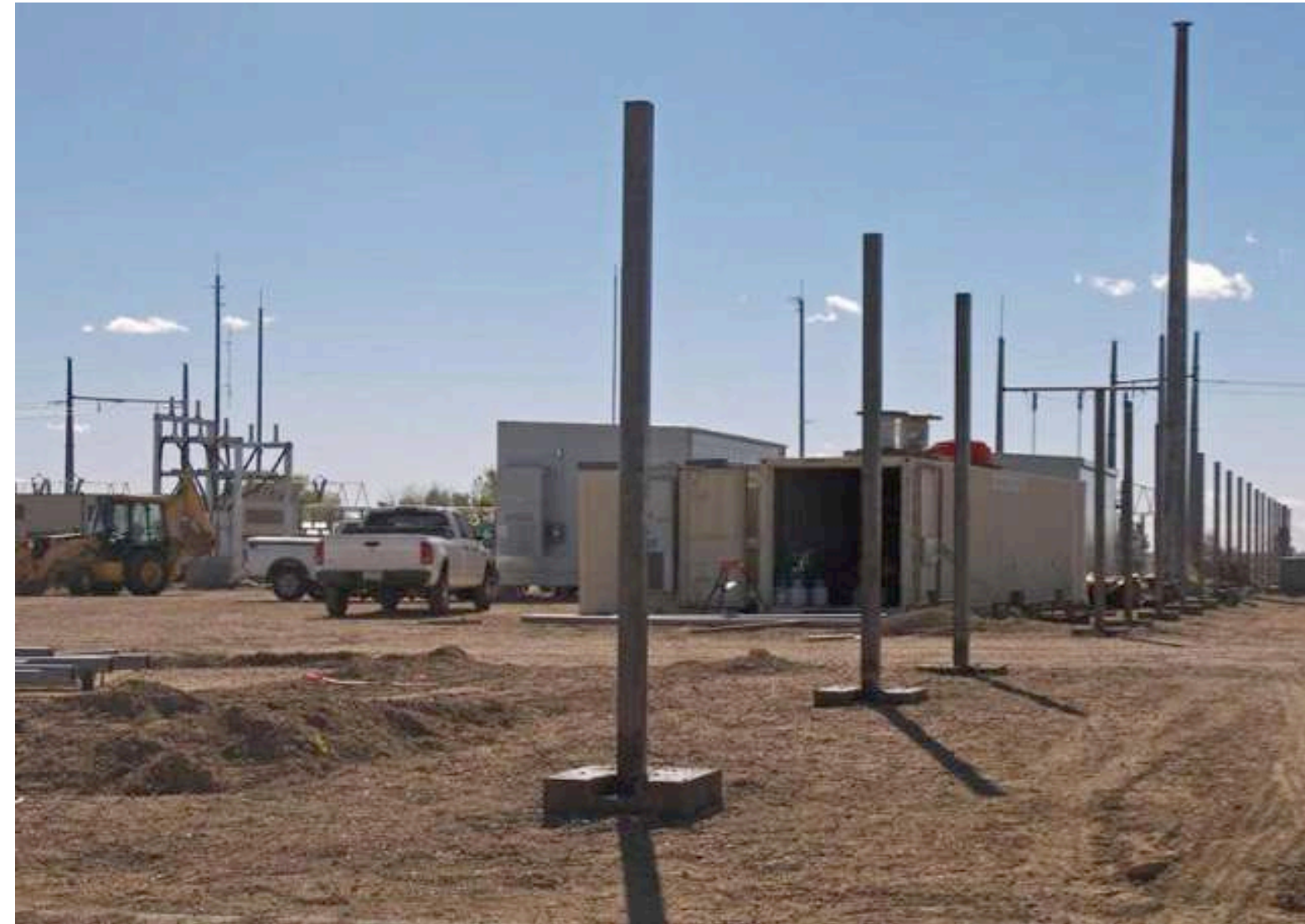
Footings with Extended Steel Supports Are Set Up for Taller Walls
